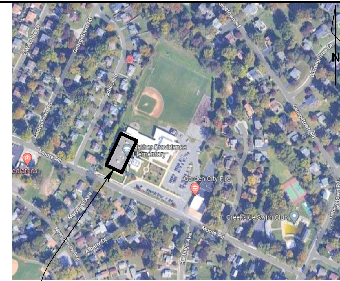
ROOF REPLACEMENT LOCATION (APPROX. 17,000 S.F.)
